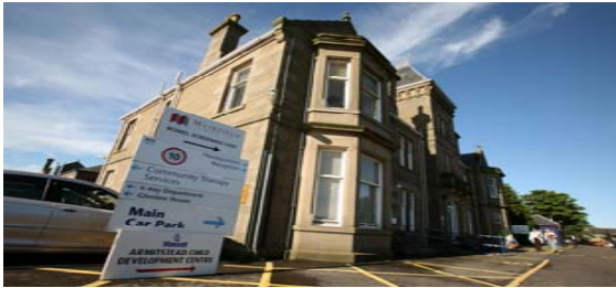
Kings Cross Hospital
